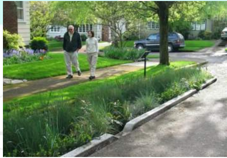
Bioswale collecting stormwater runoff
