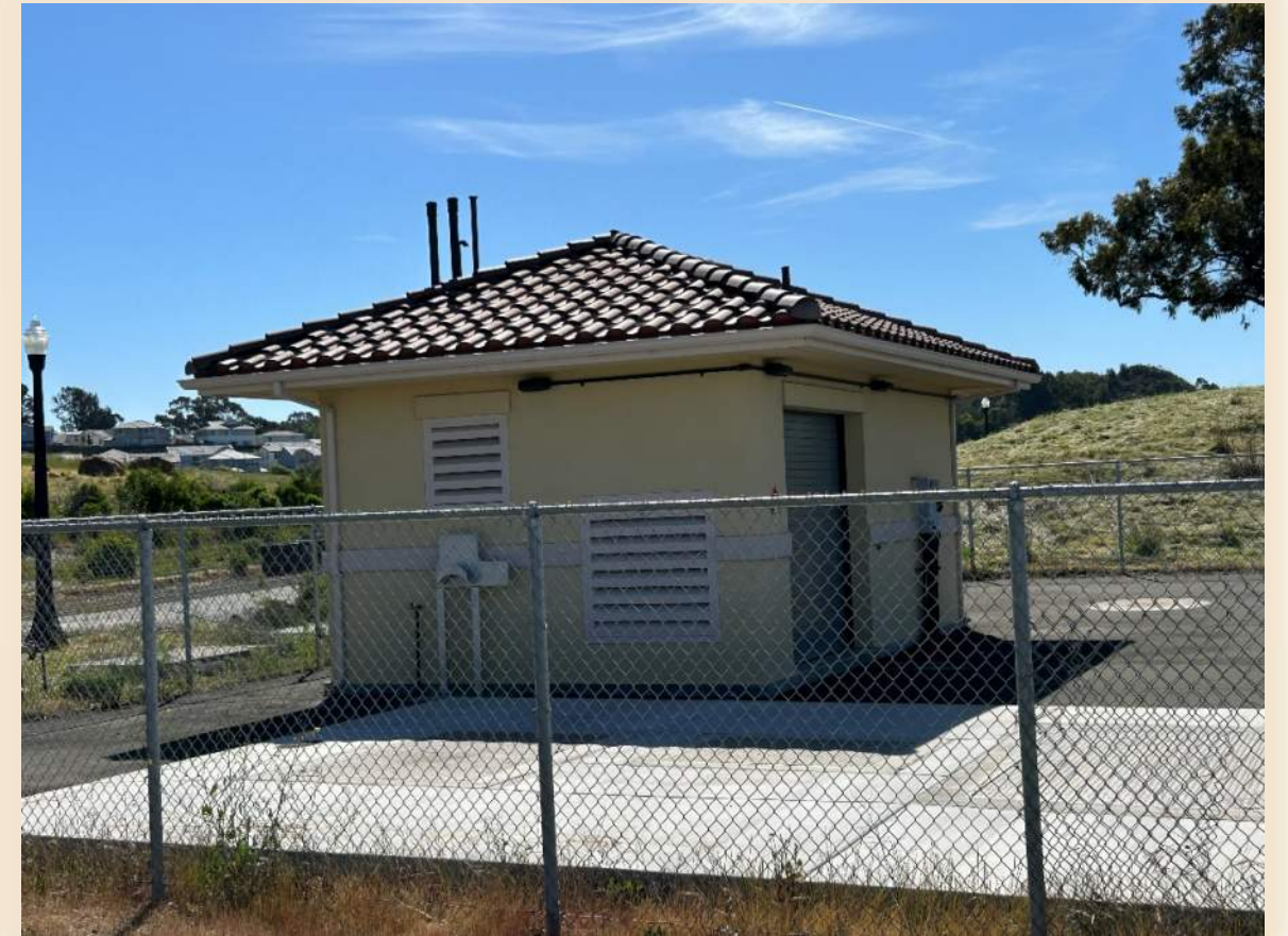
Upgraded Pump Station on Mare Island
